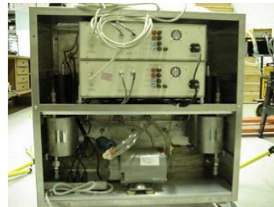
Bubblers and controls
